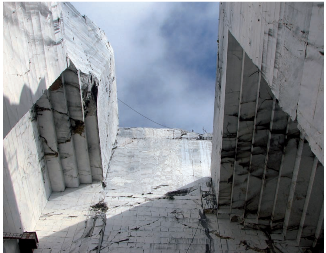
FIG. 20 - Overhanging cliff in a quarry of Carrara marble (photo E. Lotti).
